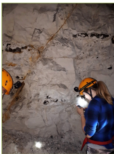
Figure 6: A fault line observed within the mine. Displacement can be seen in the offset of the flint band.
